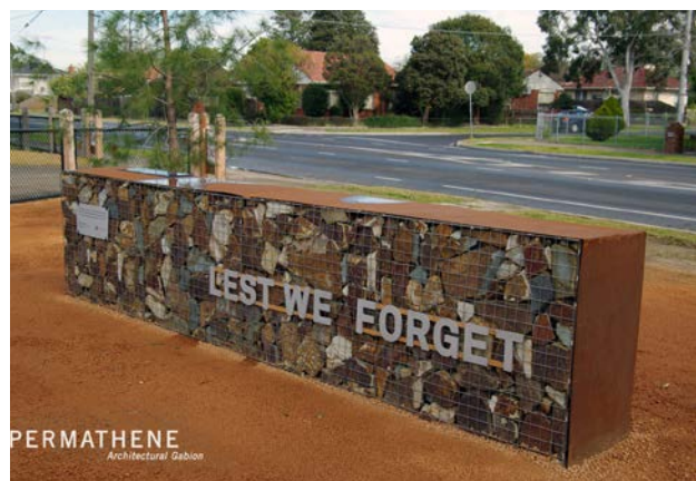
Malahang Reserve Stainless steel gabion incorporated with corten steel
