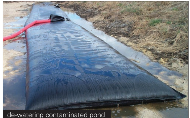
de-watering contaminated pond
