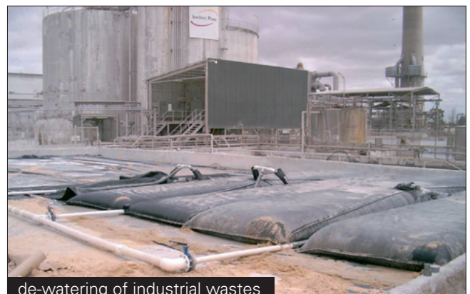
de-watering of industrial wastes
