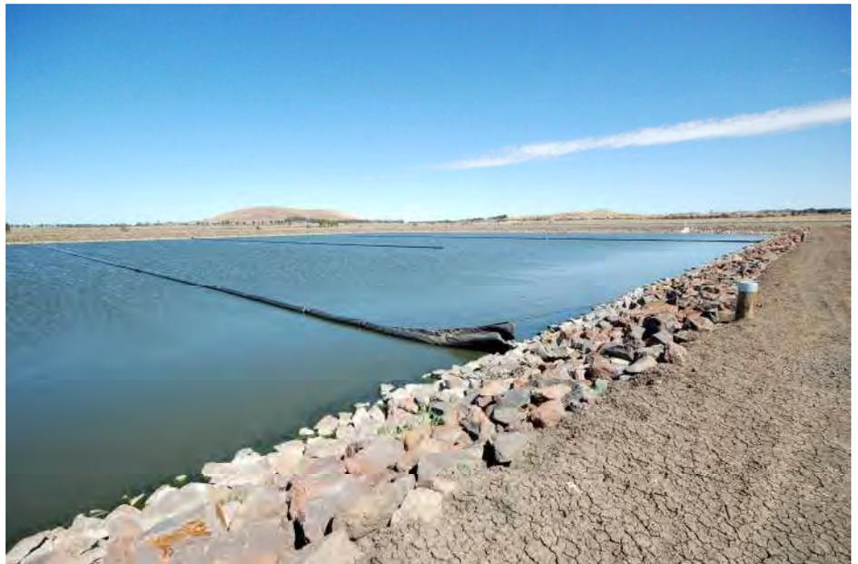
The upgrade program for the Wallan STP in Victoria, Australia, called for 3 baffle curtain to be installed in the plant's oxidation pond.
