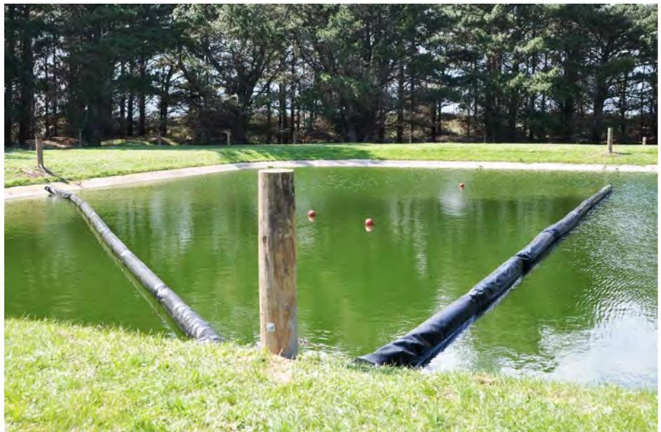
Porangahau WWTP installed three baffle curtains—one turbidity barrier to lengthen the water passage through the oxidation pond, one cut-off (shore to shore) baffle curtain with an opening to create a small maturation area around the pond's outlet, and one 4m long inlet screen
