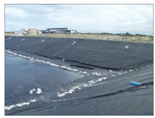
In addition to the fact that no excavating was allowed, the wetland terrain made this project exceptionally challenging, During preparation of the site, underground drains pumped water from the area to be lined and bund walls were formed. This made the site inaccessible to vehicles and a road had to be built to allow access to the area and enable installation of the liner to commence.
