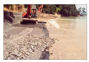
The contractor selected Syntex GHS 70/70 (70 kN x 70 kN)Woven High Strength Geotextiles based upon its excellent performance on similar projects.
