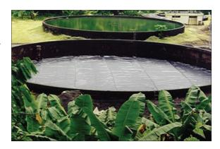
For rehabilitation of the filters, it was suggested by engineers to remove sand and wash it and prevent further infiltration of fine silt material into the lower gravel layers. To achieve this, Syntex GHS 35/35 high strength woven geotextile was recommended to be placed on top of the gravel layer because of its high strength and superior hydraulic properties.
