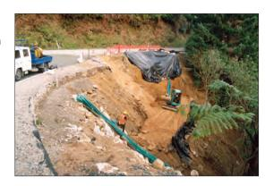
After thorough discussion with the Contractors, Syntex GHS 35/35 ( $35 \text{ kN} \times 35 \text{ kN}$ ) and GHS 70/70 ( $70 \text{ kN} \times 70 \text{ kN}$ ) High Strength Woven Geotextiles were approved for use in the construction of the Mechanical Stabilised Earth (MSE) wall.
