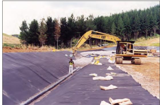
Syntex GNP E1 has been specifically designed for use in landfill or waste disposal facilities. United States Environmental Protection Agency (EPA) 9090 accelerated testing performed on this product has demonstrated an excellent chemical compatibility with landfill leachate. It is highly resistant to puncture, impact and abrasion, which greatly reduces the potential damage from sharp objects during and long after the construction process.
