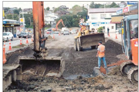
Syntex GNP A1 (Strength Class A) nonwoven, needlepunched, staple fibre geotextile was used as the lightweight subgrade separation fabric to improve bearing capacity.
